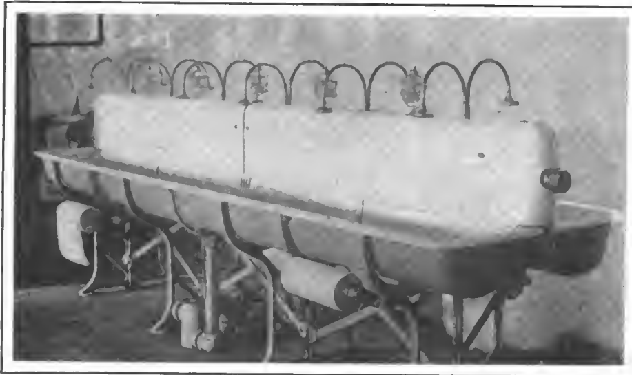
A special model unit stand where workers wash with constantly flowing non-scalding water. It was designed to eliminate the use of the wash basin and its dangers of infection.
